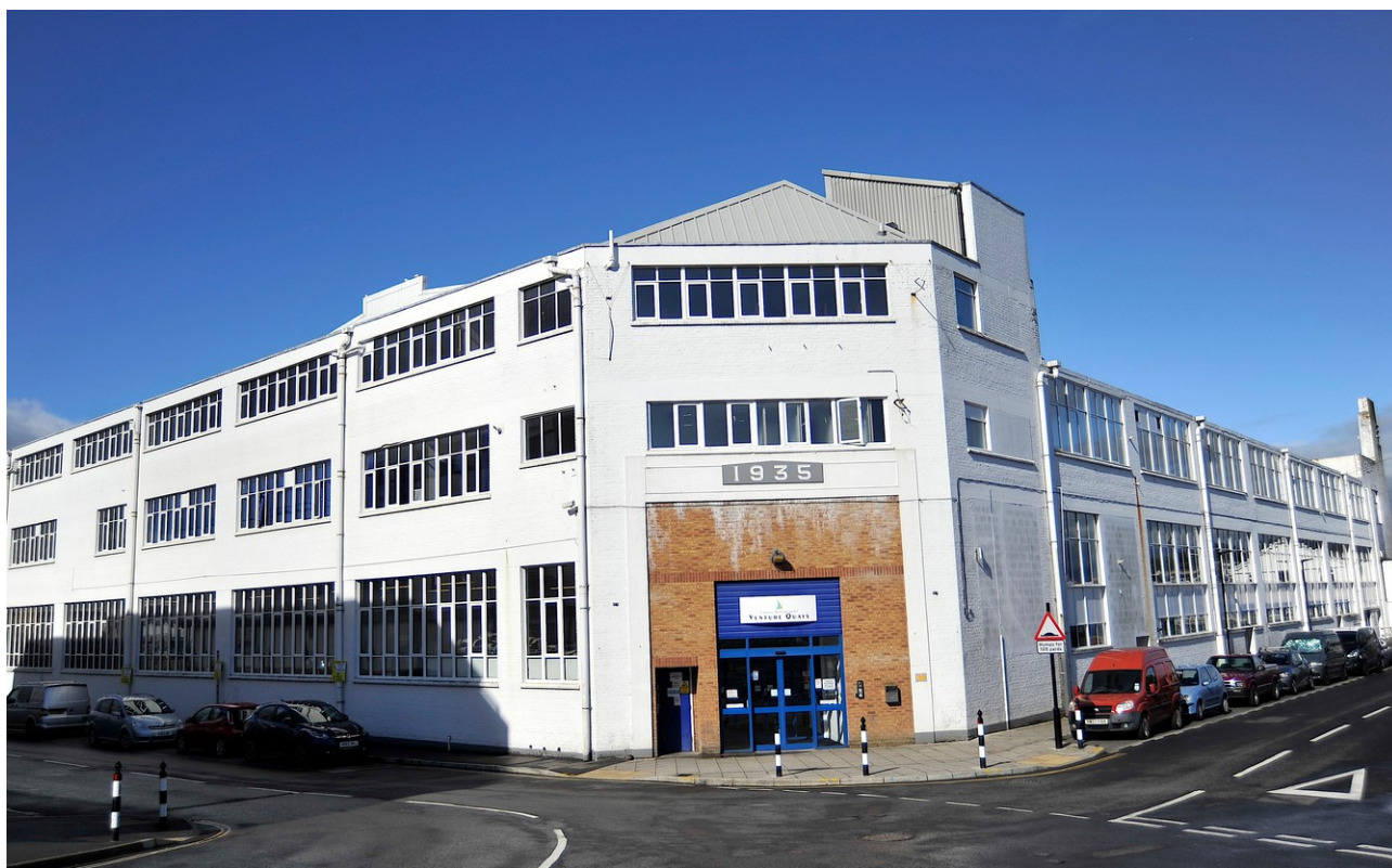
Figure 8: The local authority is now the owner of vacant office and warehouse space in East Cowes. Photo courtesy of Michael Paler
