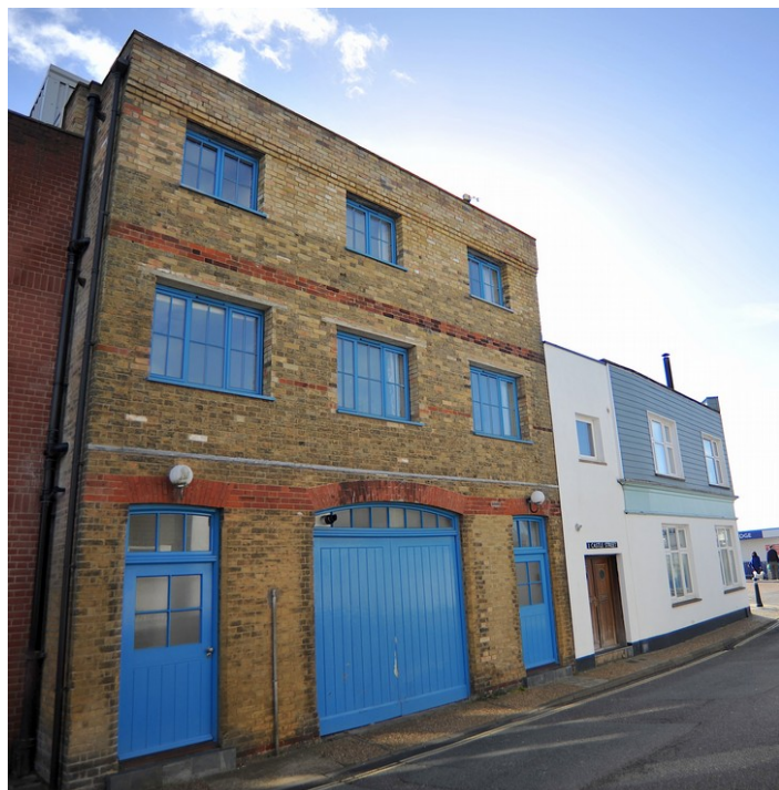
Figure 7: East Cowes town centre is the only location on the Island with a significant quantity of commercial buildings near a vehicle ferry. Photo courtesy of Michael Paler
